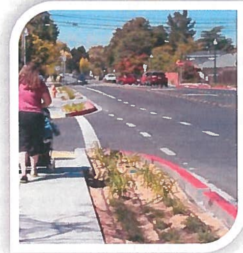
This Sustainable Street in City of San Mateo incorporates a bicycle lane and a "bioretention area" or rain garden that removes pollutants from stormwater runoff (Source: SMCWPPP).
