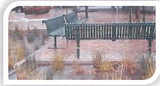
Green stormwater infrastructure is designed to mimic natural processes. This photo shows how landscaped bioretention areas help to detain and slow the flow of stormwater runoff to the storm drain system (Source: Nevue Ngan).
