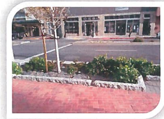
This bioretention facility in Oakland receives stormwater runoff from both the roadway and an adjacent plaza (Source: Horizon)
