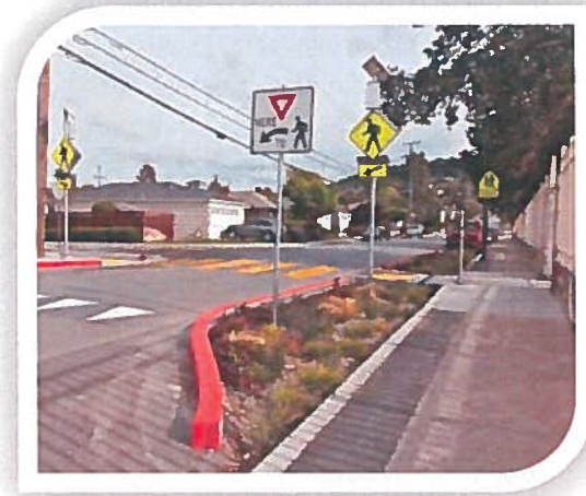
Sustainable Street in the City of San Mateo; stormwater runoff flows into a “bioretention area” or rain garden that reduces the crossing length for pedestrians near a local school (Source: SMCWPPP).
