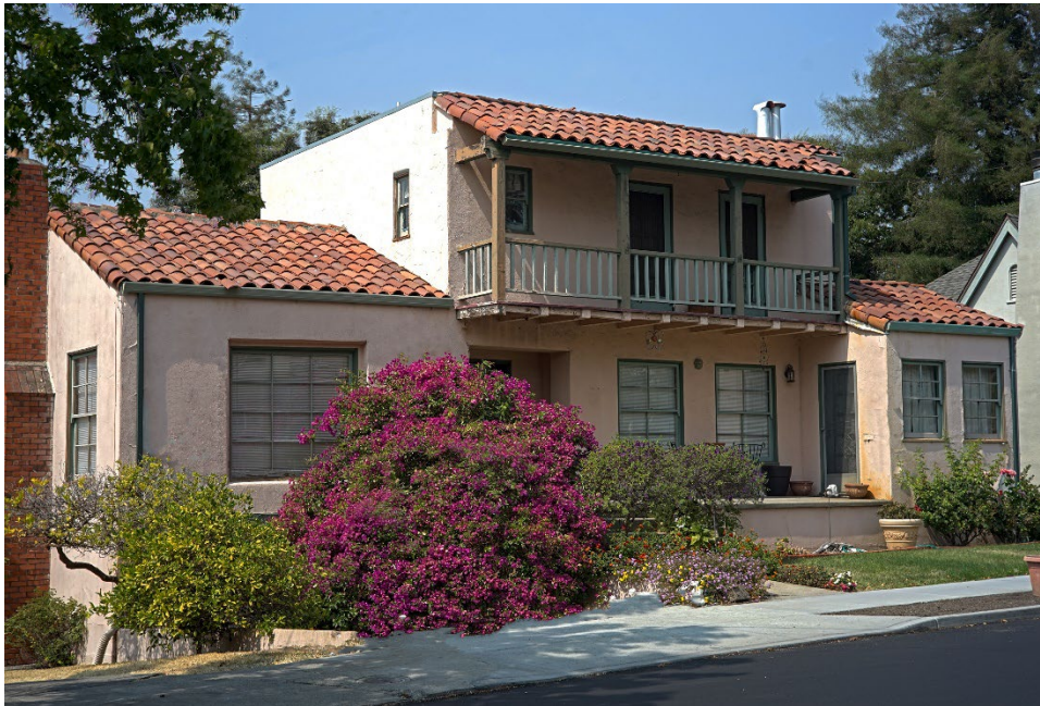
Single-Family Home on Brown Street (Source: Kevin Murray)
