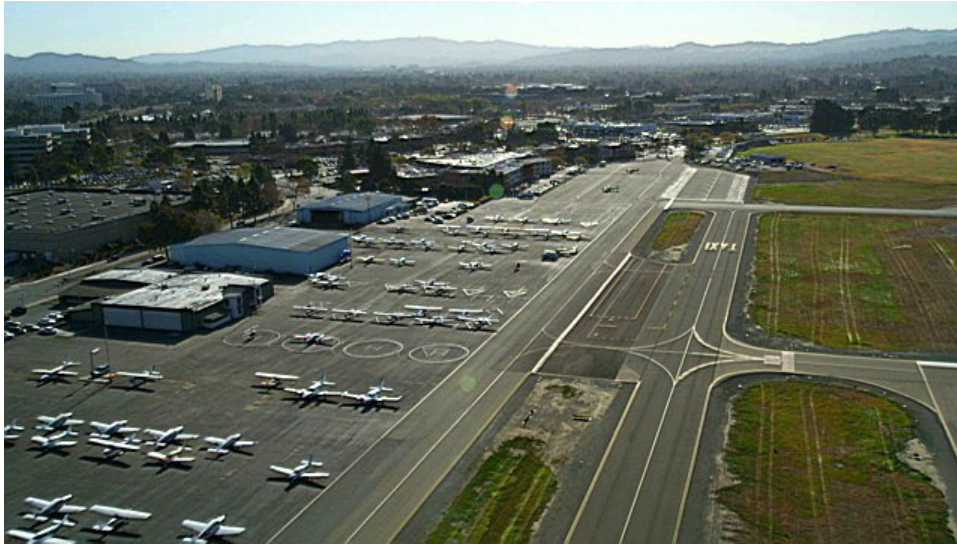
Buchanan Field Airport Runway (Source: Inspection Services Inc.)
