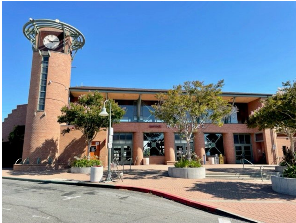
Martinez Intermodal Train Station
